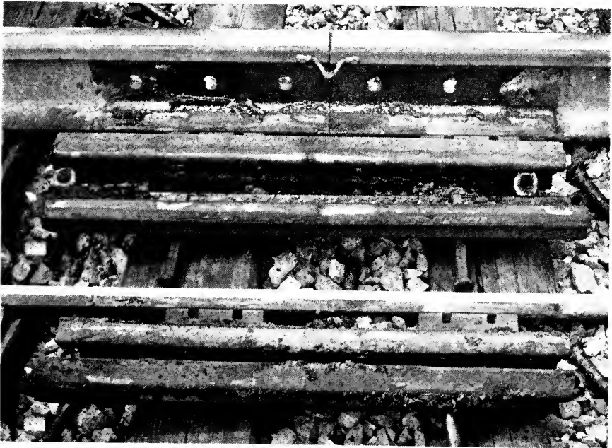
Fig. 13. Section 8, Packed with Petrolatum (Dark) and Plastic H End Plugs
